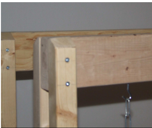
Step 8: Legs fastened to crossbeam
