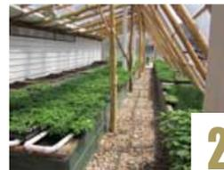
This passive solar greenhouse was designed to use as little fossil fuel energy as possible. The 56° angle of the southern face and the building's orientation at 2° east of south provide maximum solar gain during
